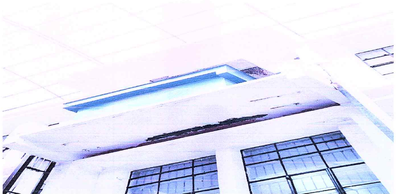
Major Repairs work required for cantilever slab below water tank in front of Library
